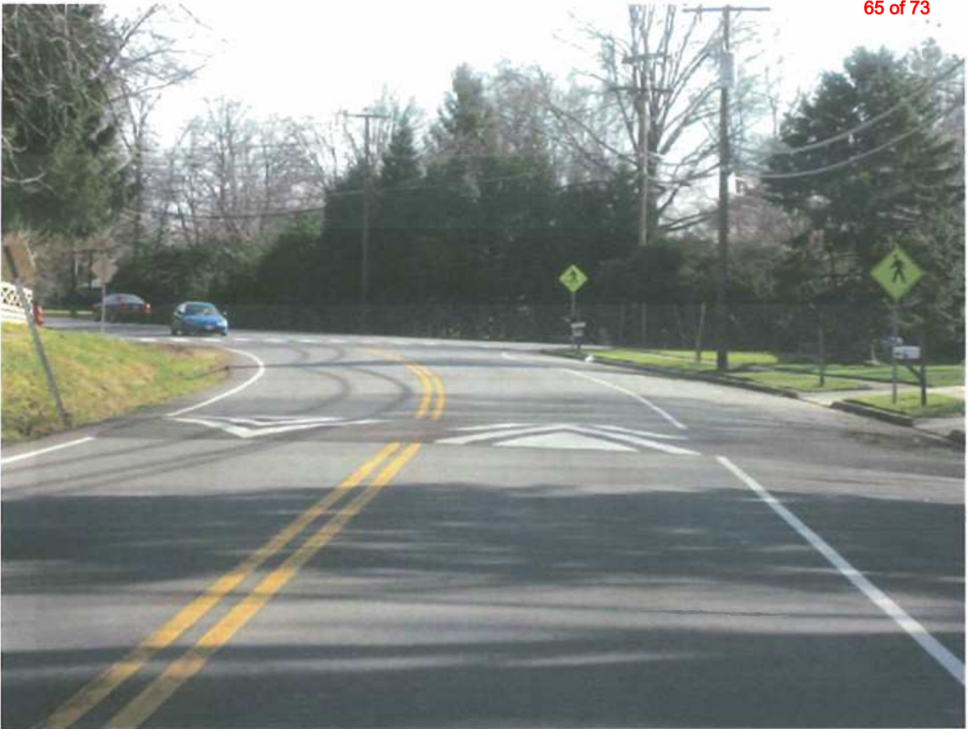
Figure 3.10.3. Speed Hump Along Horizontal Curve (Source: Scott Wainwright)
