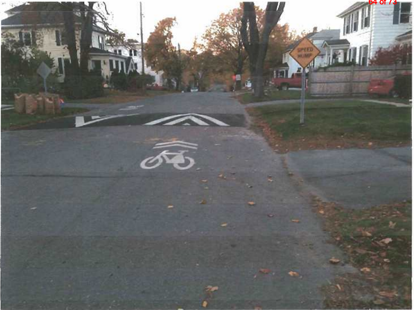
Figure 3.10.2. Speed Hump on Residential Neighborhood Street (Source: Lucy Gibson)
