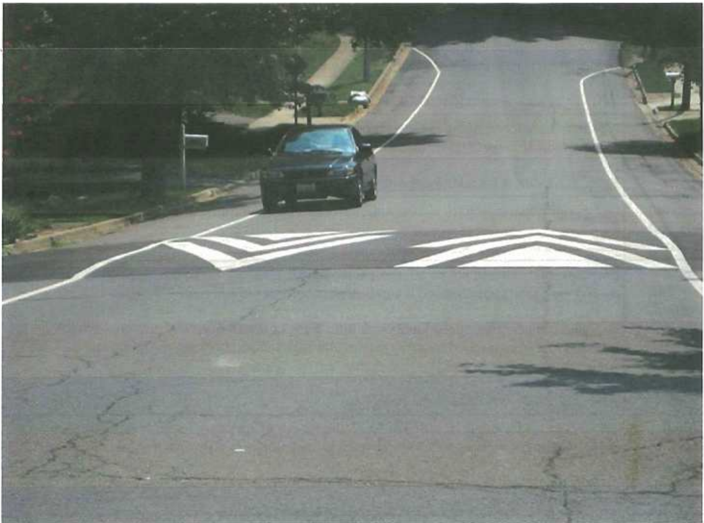
Figure 3.10.4. Speed Hump on a Grade (Source: Scott Wainwright)
